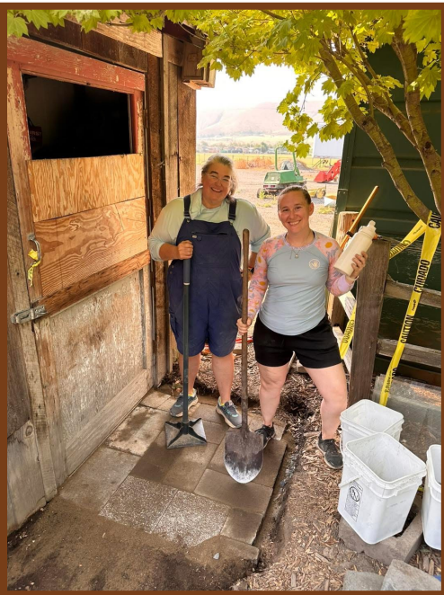
Kelly K and Mikki dug, leveled the ground, and placed pavers to smooth out the apron in front of the tool shed.
